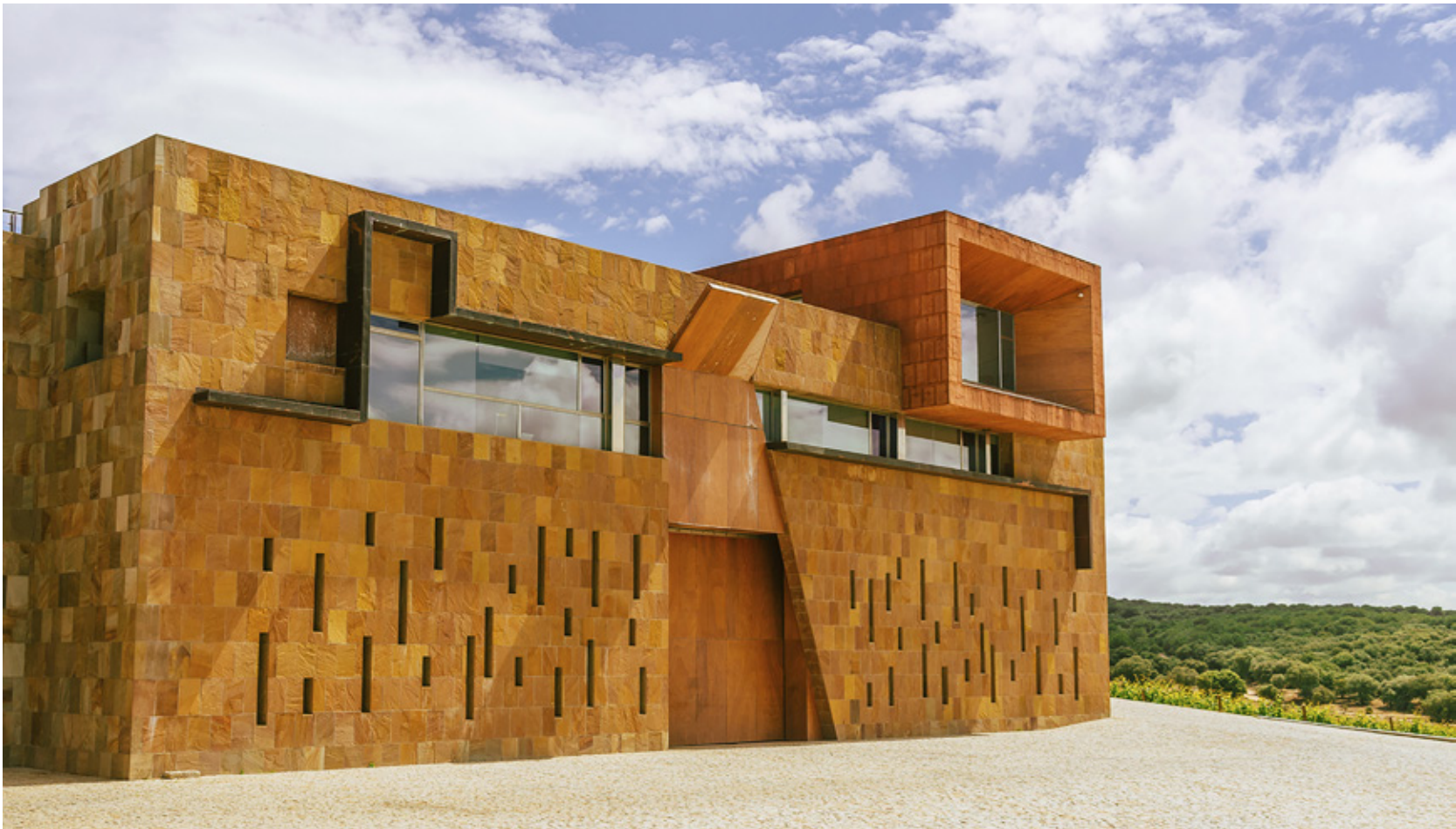
Vanguardista y original bodega | Avant-garde and original winery
