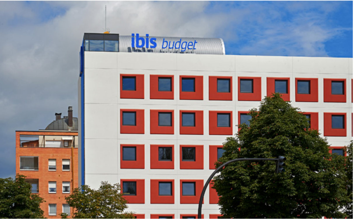
La fachada del hotel se ha diseñado pensando en la eficiencia energética / The façade of the hotel has been designed with energy efficiency in mind
