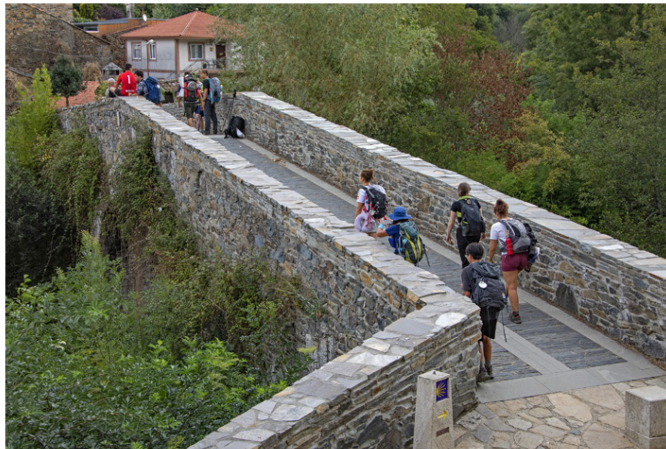
Medieval bridge of Furelos, Melide | Puente medieval de Furelos, Melide
