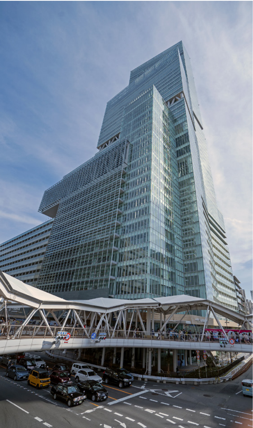
Edificio Abeno Harukas | Abeno Harukas Building
