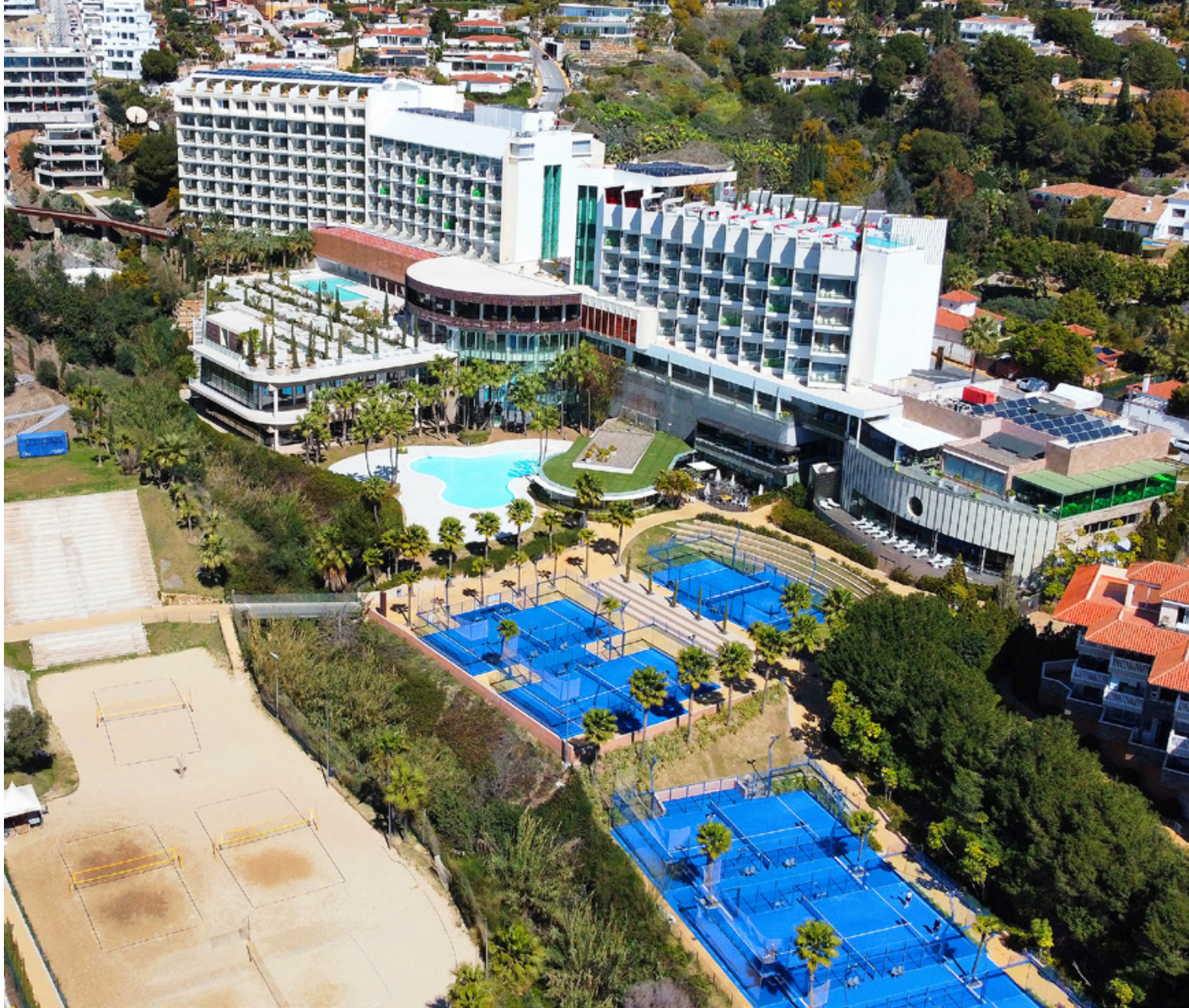
Hotel, facilities and sports courts at Higuero Resort | Hotel, instalaciones y pistas deportivas de Higuero Resort
