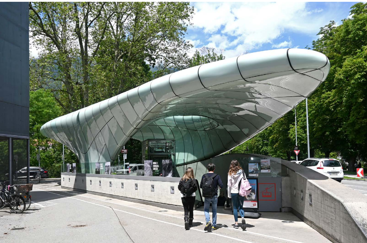
Futuristic access to the Nordkettenbahn funicular railway / Futurista acceso al funicular de Nordkettenbahnen
