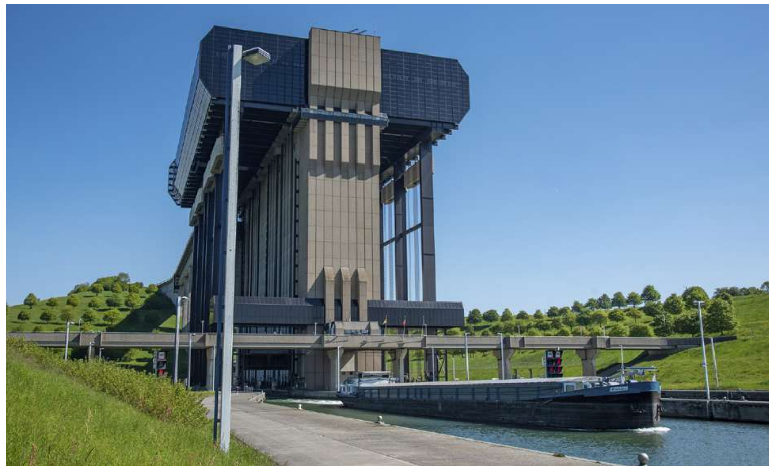
Gran Canal du Centre | Main Canal in the Centre
